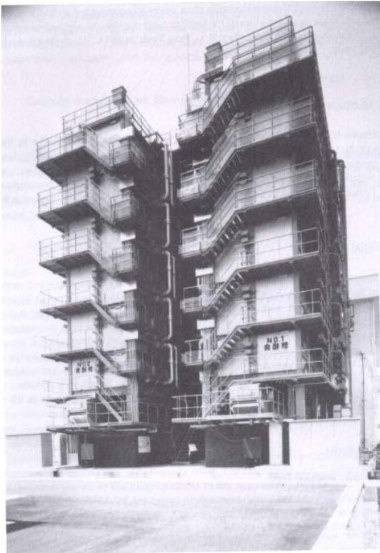
**Fig. 4 - NGK vertical, multistage, agitated bed-composting system (Haug, 1993)**
