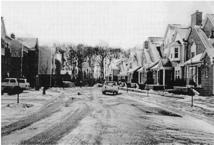
FIGURE 2 A residential street within Main Street Village.
