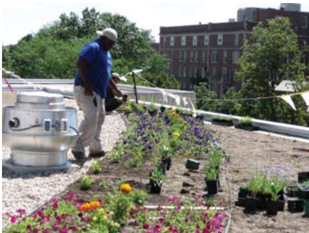
Planting the new green roof on Sandburg Commons.
