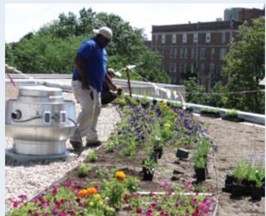
Planting the new green roof on Sandburg Commons
